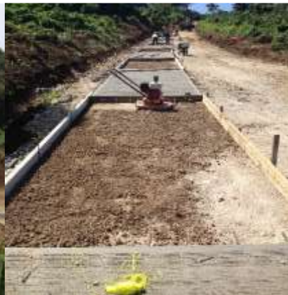
Gravelling- ripping, pack filing and compacting
