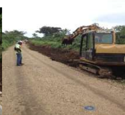
Formations/ Preparations- concrete pavement bays @ 5m X 2m X 0.15m
