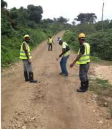
Setting out- centerline, road widths and shoulders to drainage
