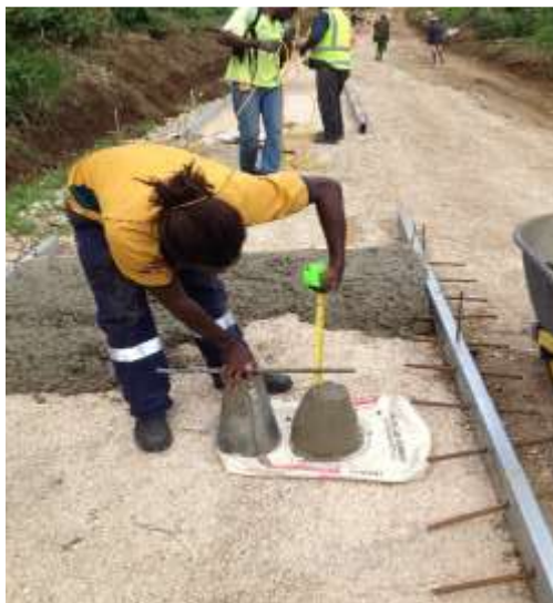
Concrete slump test
