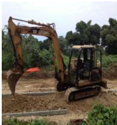
Gravelling- ripping, pack filing and compacting
